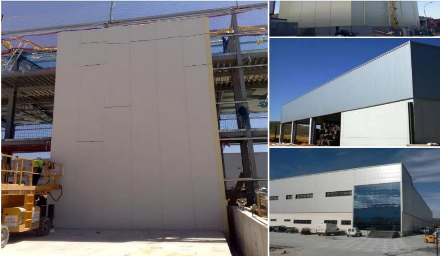
Warehouse Built With Aistein Panels
